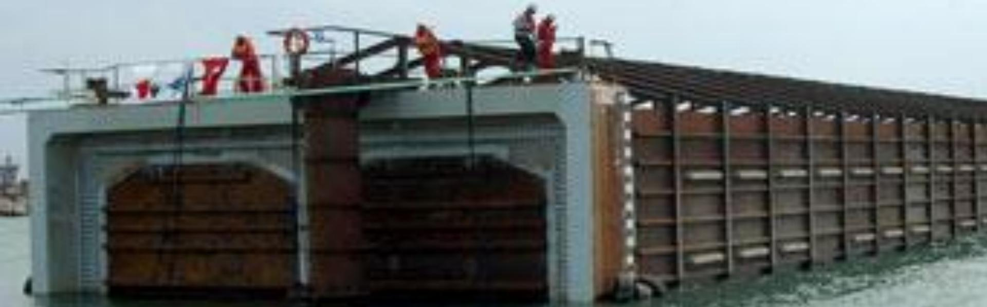
*The floating tunnel segment is towed close to the previously installed*
